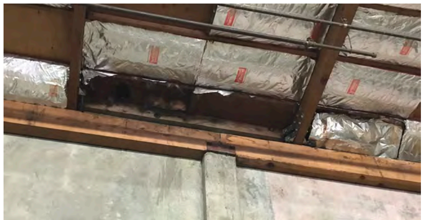
Retrofit roof-to-wall anchors – east wall
