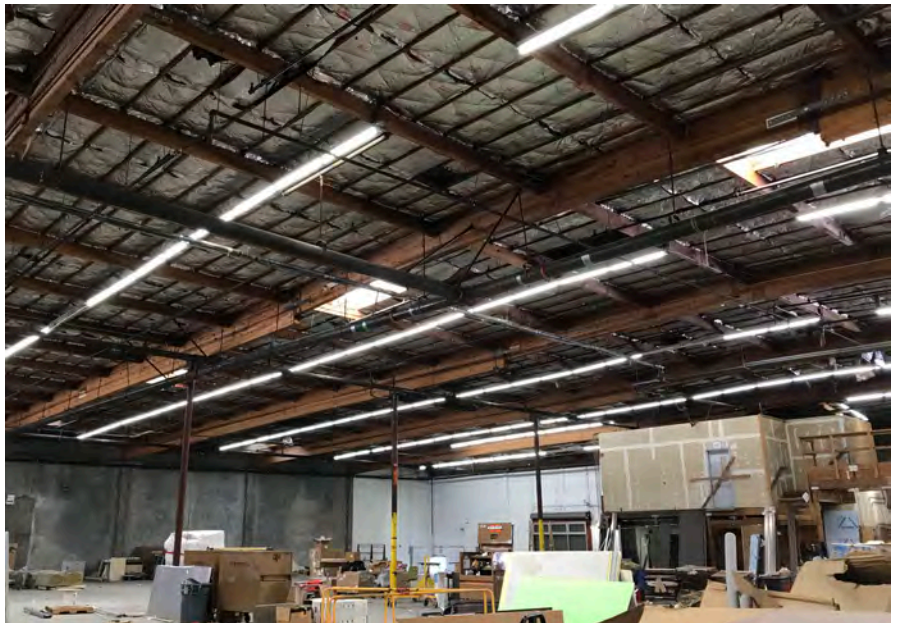
Warehouse - looking toward southwest corner
