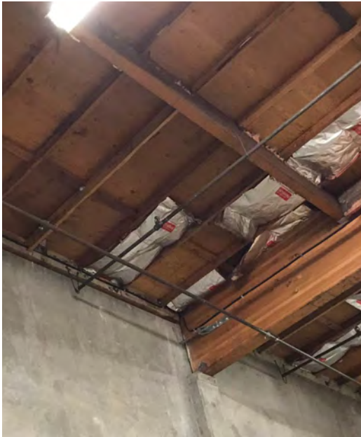
Retrofit roof-to-wall anchors – north wall
